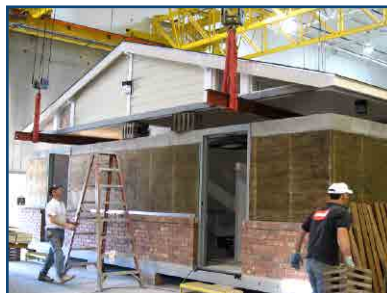
7 | Roof is Installed on CMU Walls
