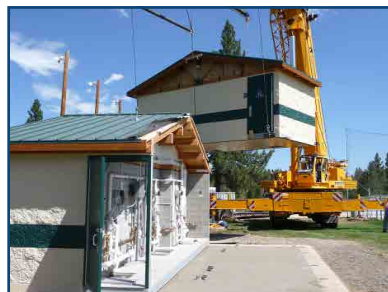
10 | Drop-In-Place Installation with a Crane
