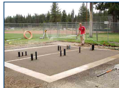
9 | Sub-Grade Pad Preparation
