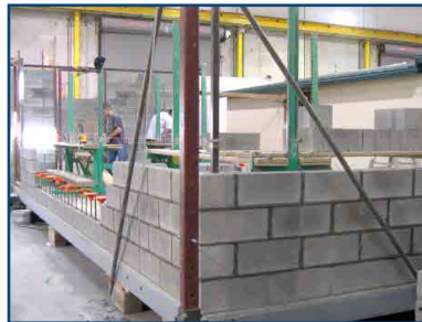
5 | CMU Walls Constructed on Concrete Slab
