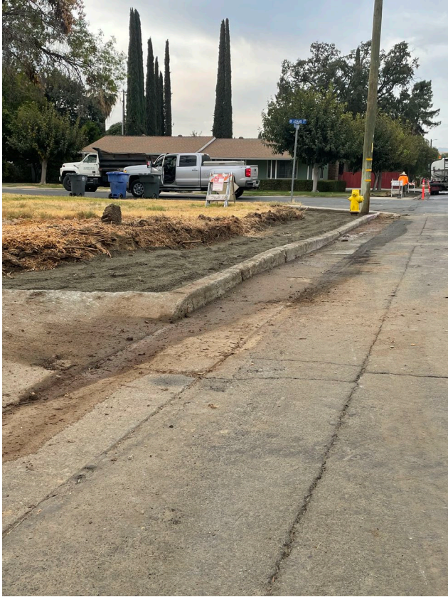
Extra Demolition Limits to Match clean edge
