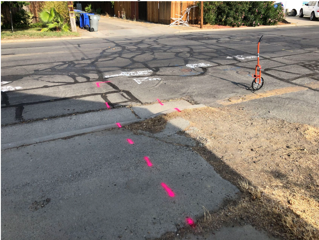
Extra Demolition Limits to Match clean edge
