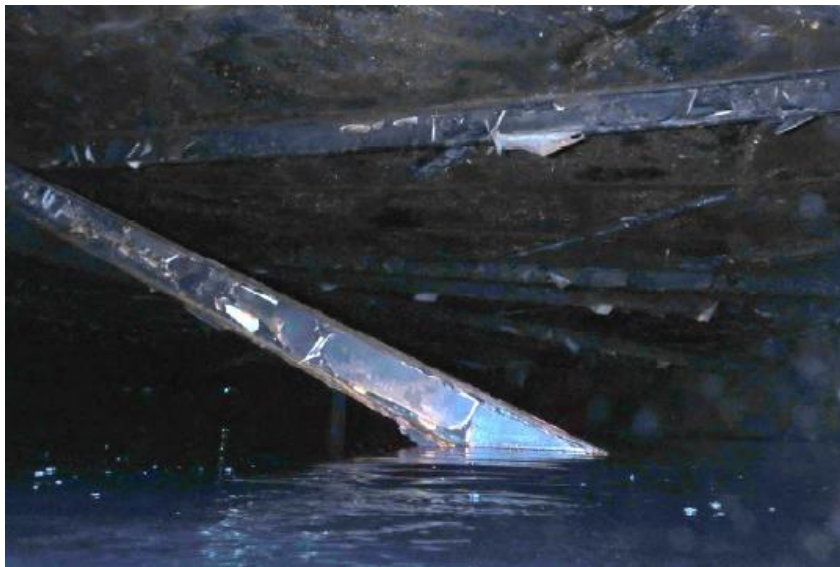
Figure 9: Failing Fixed Roof Rafters (By CSI on 01/06/20)
