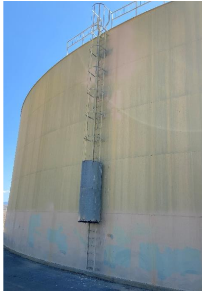
Figure 10: External Access Ladder (By MKN on 04/21/21)
