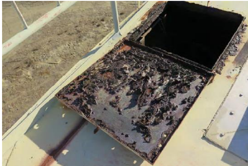
Figure 3: Corrosion at Roof Hatch (By CSI on 01/06/20)
