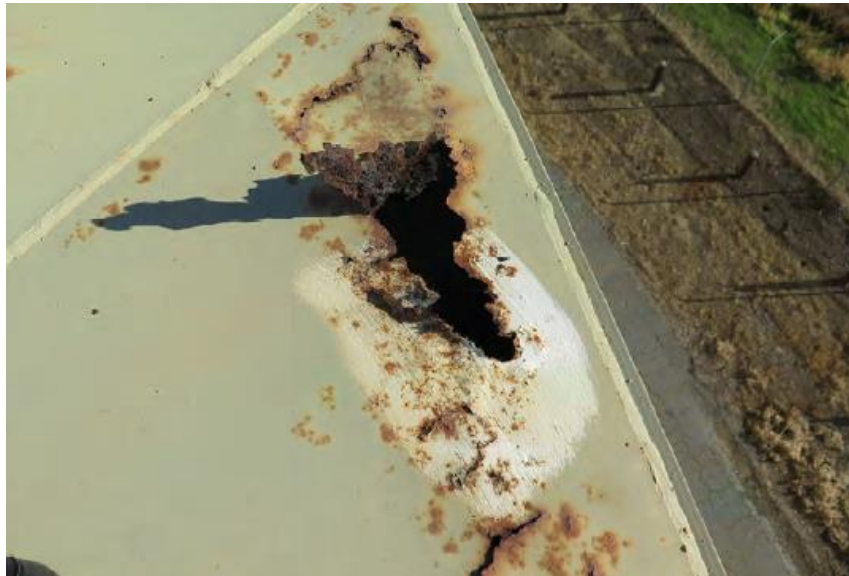
Figure 8: Fixed Roof Exterior Corrosion (By CSI on 01/06/20)
