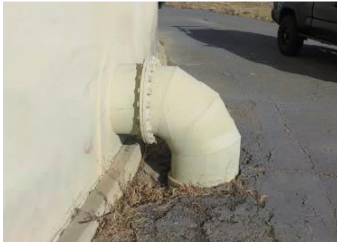
Figure 14: Overflow Pipe (By CSI on 01/06/20)
