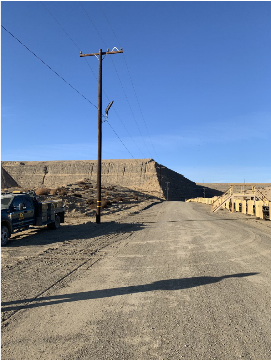
Power for conveyors will be supported by power poles to be installed approximately every 250' along beltline. Power poles will be 35' tall (45' long with 10' driven into the ground). The power poles will have LED lighting fixed to poles, placed about 25' above grade.
