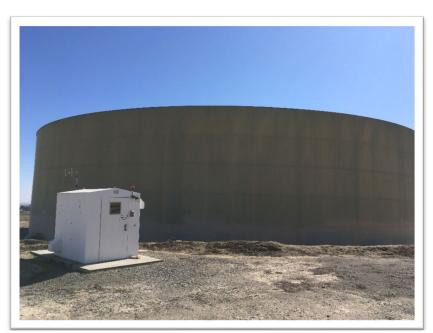
The Derrick Avenue Reservoir has capacity for 7.6 million gallons. It is the City's largest and primary storage tank and delivers drinking water into the city limits. The steel tank is nearing the end of its useful life due to corrosion.
