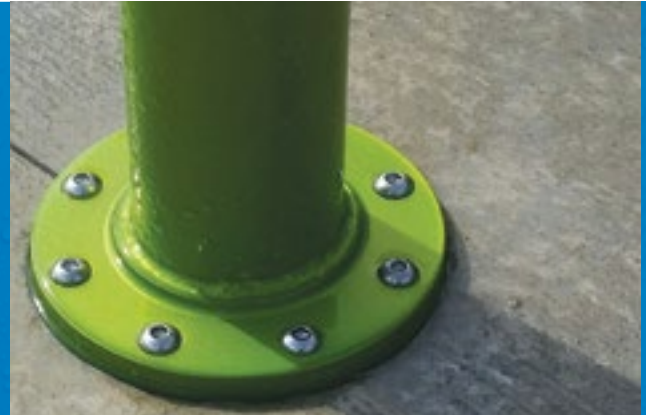
STAINLESS STEEL FOOTING BASE INSTALLATION
